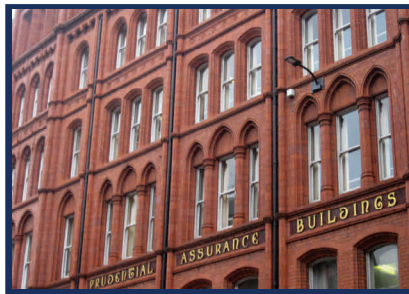
Picture - Prudential Assurance Building, Liverpool, designed by Liverpool architect Alfred Waterhouse, also noted for their Holborn, London office and the Natural History Museum, and whose brothers were founding partners of accountants PricewaterhouseCoopers and solicitors Field Fisher Waterhouse.
